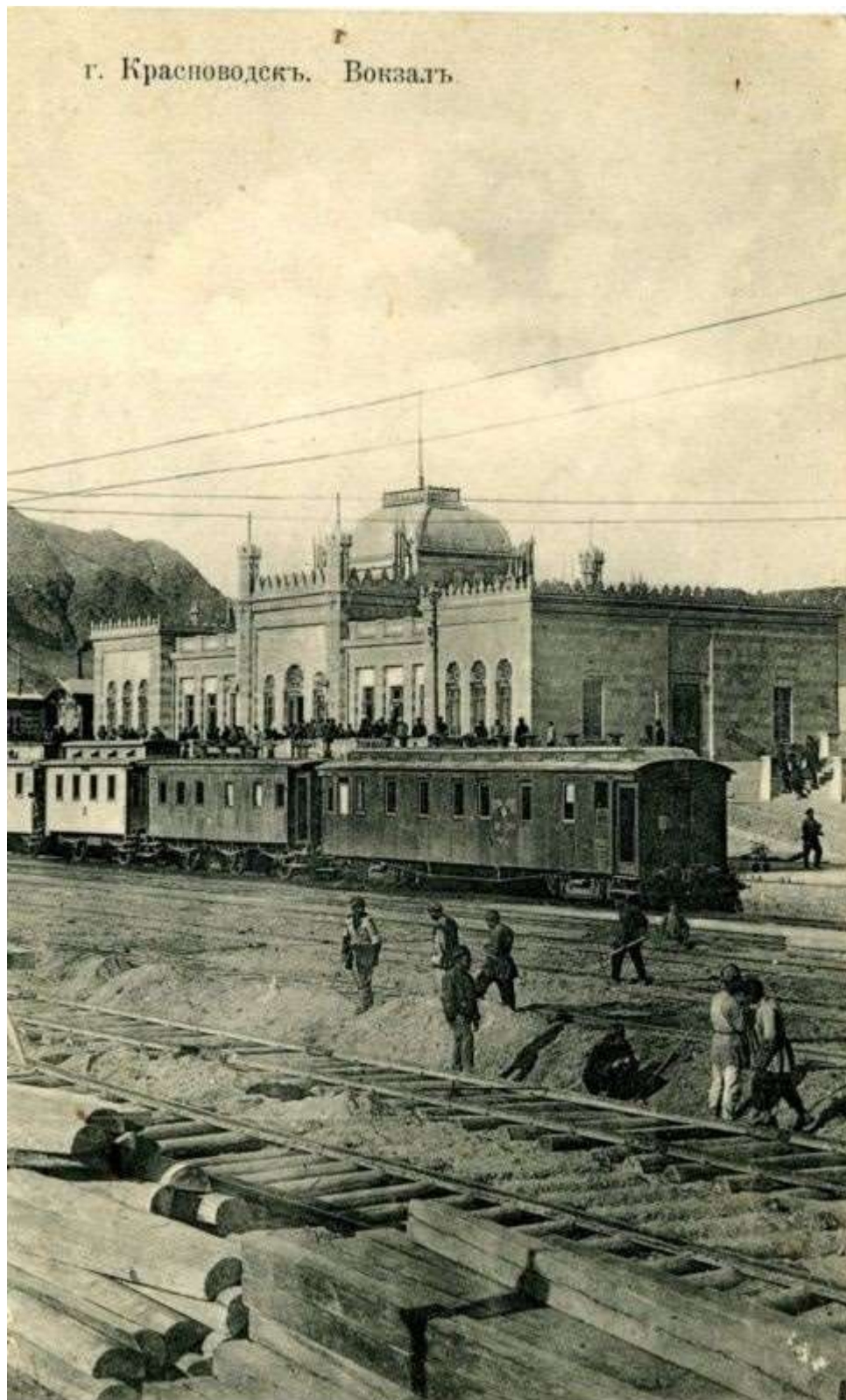
Trans-Caspian railway station at Krasnovodsk (currently Turkmenbashi)
