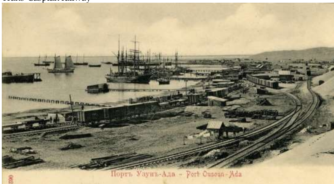
Trans-Caspian railway station at Uzun Ada ('Big Island') port
